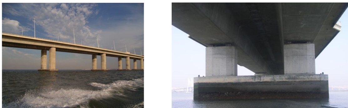
Figure 2.7. General view of the central viaduct (left) and view of the tidal zone of a prefabricated caisson (right)
