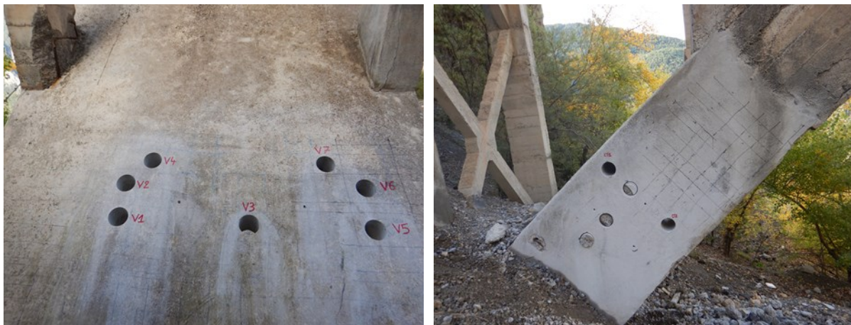
Figure 2.75. Cores taken on the springing of the arch on the left bank (photo on the left) and in the arch rib on the left bank, upstream (photo on the right)
