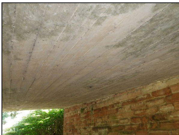
Figure 2.65. Intrados of the deck on the right bank abutment side.
