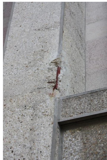
Figure 2.88. Localized spalling on a corner at the location of an old repair
