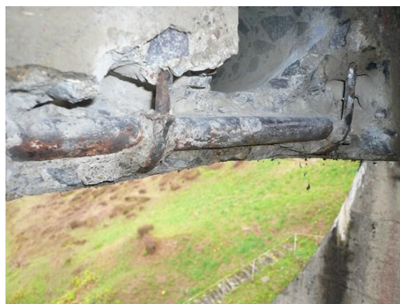
Figure 2.99. Autopsy of a beam heel showing a surface oxidation of the longitudinal and transverse reinforcement
