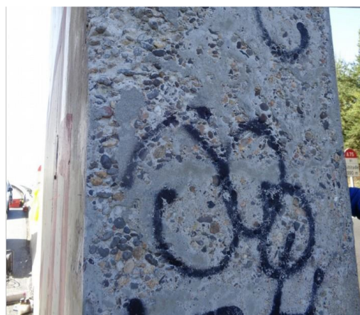
Figure 2.58. Scaling of concrete
