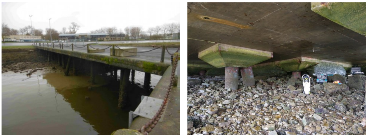
Figure 2.34. Left: View of the TCD wharf on the Scorff channel; Right: Capitals on inclined piles
