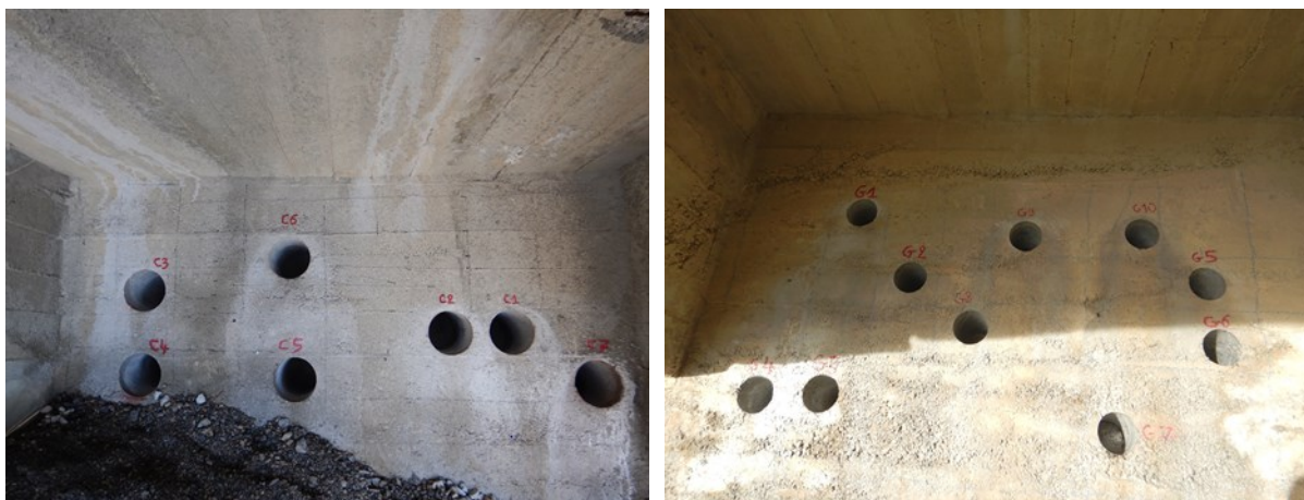
Figure 2.76. Cores taken in the massive blocks at the foot of the arch respectively on the left bank and on the right bank (respectively photo on the left and on the right)
