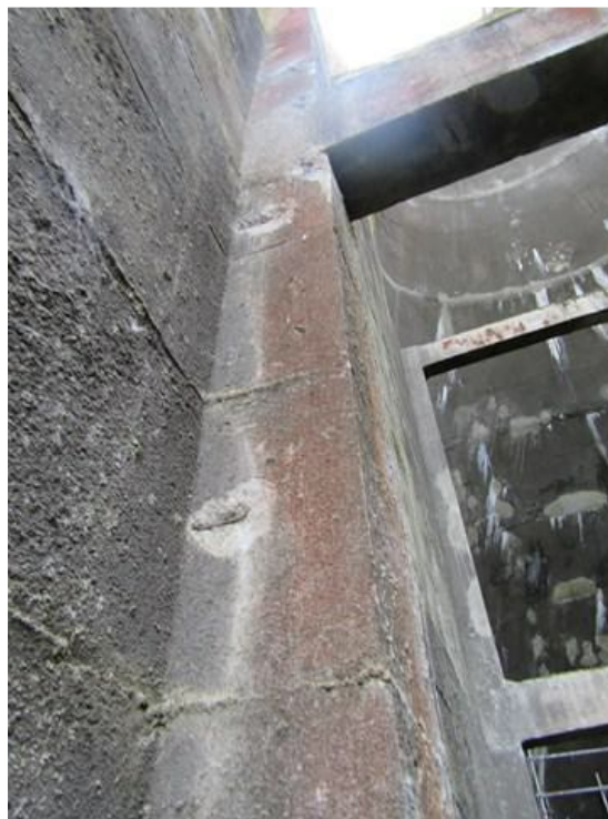
Figure 2.97. Concrete spalls on a buttress
