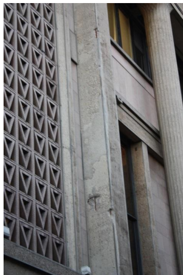
Figure 2.87. Spalling at the edges with apparent steels
