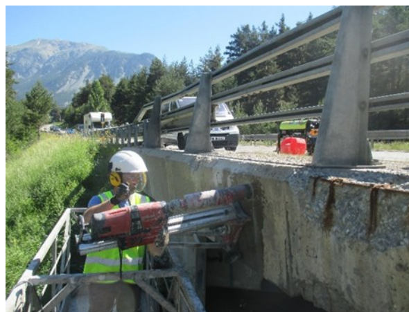
Figure 2.48. Coring on the upstream cornice
