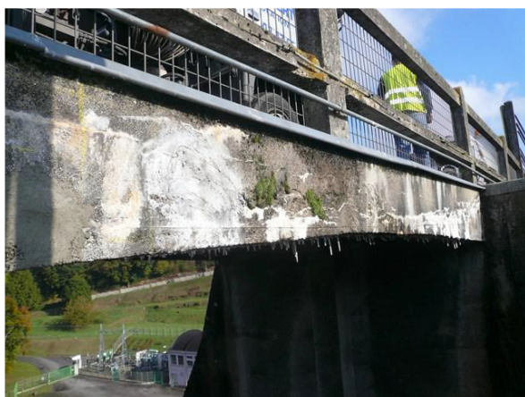
Figure 2.98. Longitudinal cracking (with calcite) of an edge beam (upstream web) of the deck
