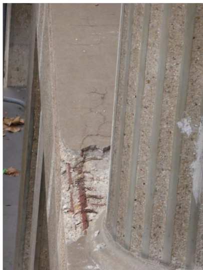
Figure 2.86. Spalling on a horizontal surface revealing the corroded reinforcements
