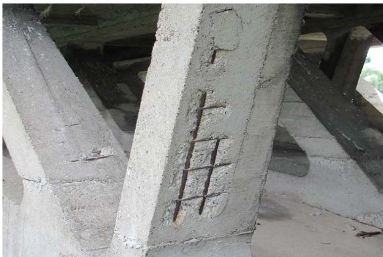
Figure 2.79. Localized concrete spalling on a diagonal due to an insufficient cover
