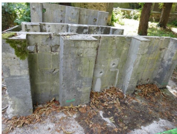
Figure 2.91. Slab A with drilling area of cores 1 and 2. Internal face
