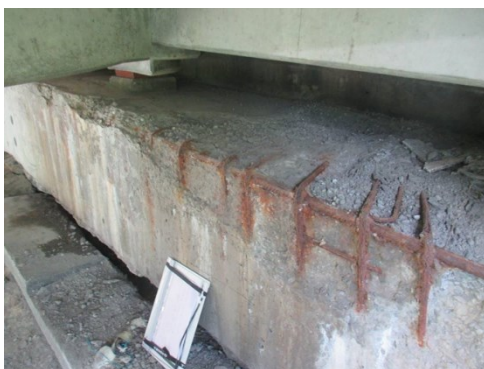
Figure 2.45. Spalling of concrete of the capbeam (C0 abutment)
