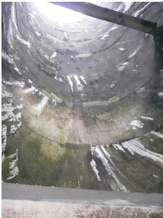
Figure 2.96. Presence of leakage with calcite in the vault between the cold joints
