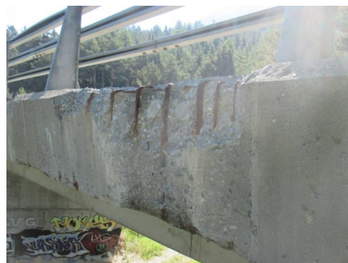
Figure 2.46. Exposed corroded steels, concrete spalling on the cornices
