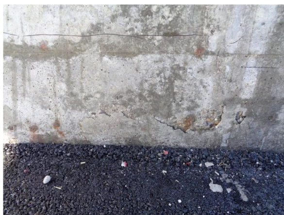
Figure 2.57. Spalling of concrete with traces of oxidation
